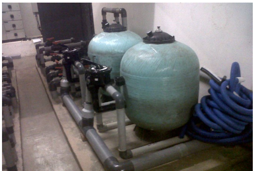
Filter Plant Installation
